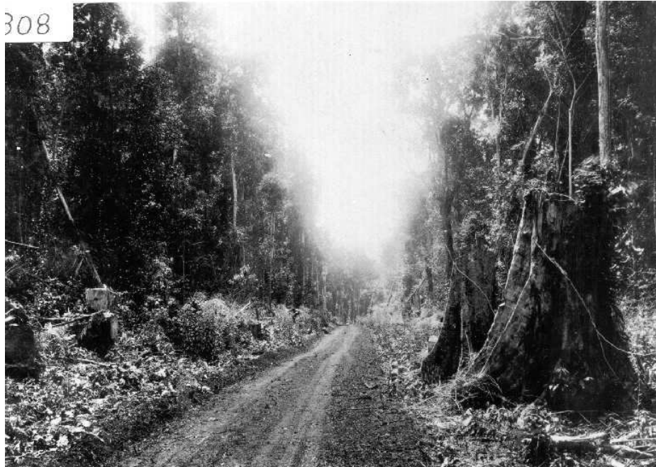
The Mission Beach - El Arish Road under construction in the 1930's
