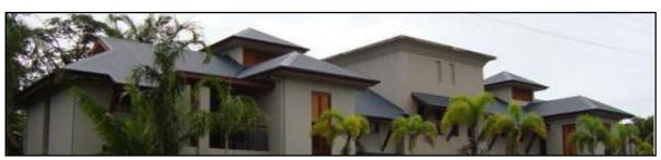
This roof design provides a good example of the use of large eaves and a staggered roof profile to break up the bulk of the roof. The roof is also constructed using Colorbond sheeting.
