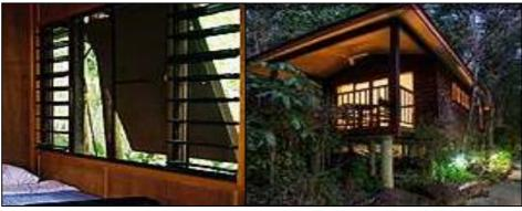
Example of awnings comprised of timber battens to encourage shade and protect openings (*Images sourced from:*
