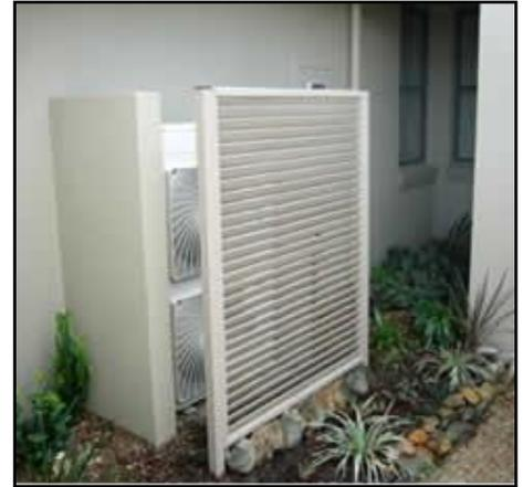
An example of an air-conditioning screen located at ground level
