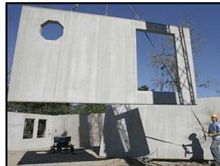
Prefabricated Concrete Panel
