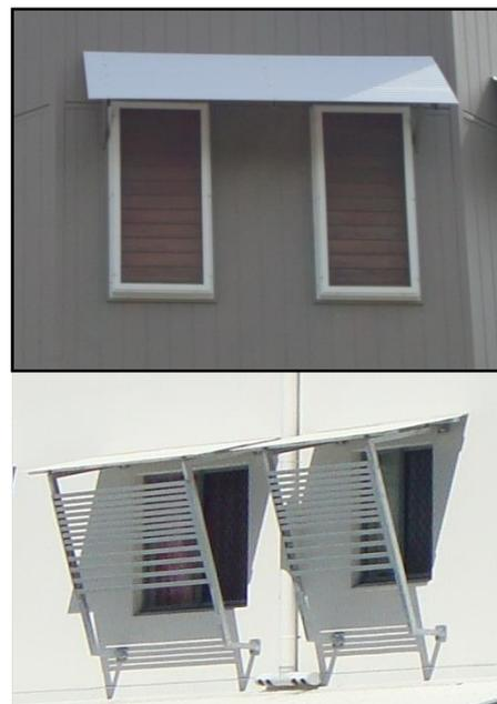
An example of louvres that are designed for tropical climates being shaded by an awning
