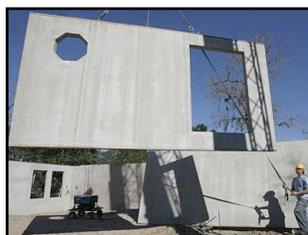
Prefabricated Concrete Panel
