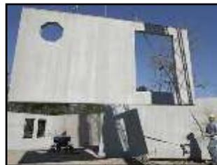
Prefabricated Concrete Panel
