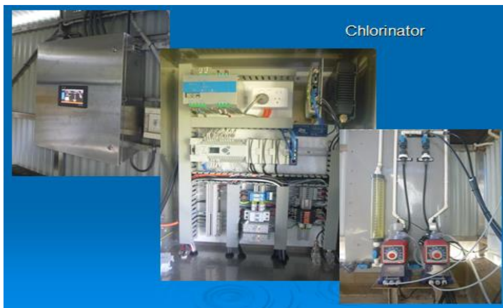
Figure 5.6: Facilities at the Bulgun Ck Chlorinator - SCADA and dual dosing pumps.
