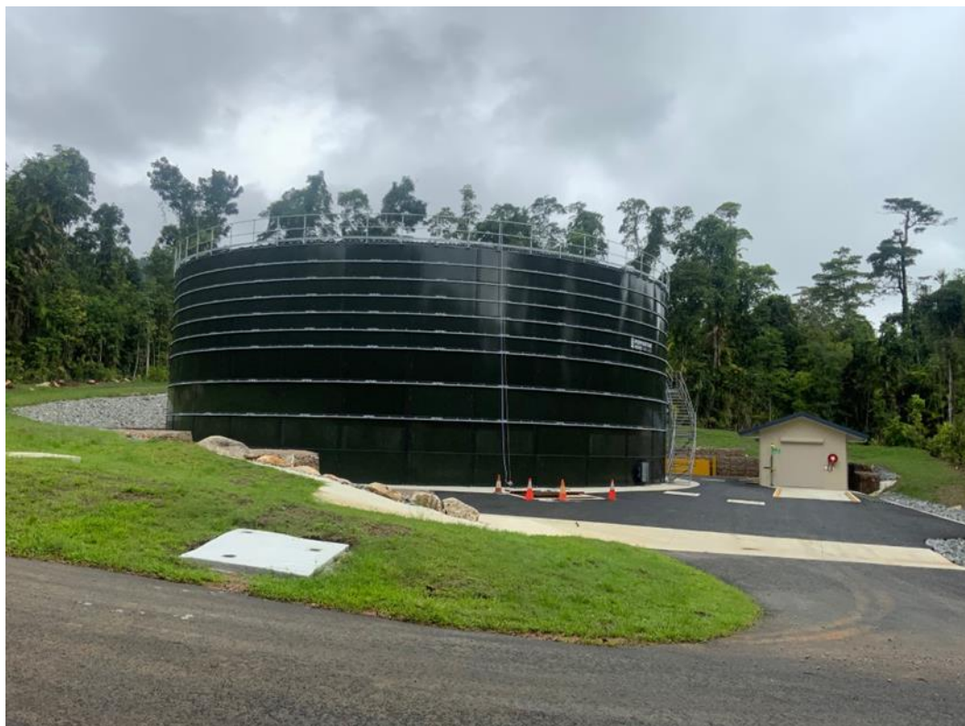
Figure 5.1: 4.5 MI Bulgun intake reservoir and Chlorine dosing building
