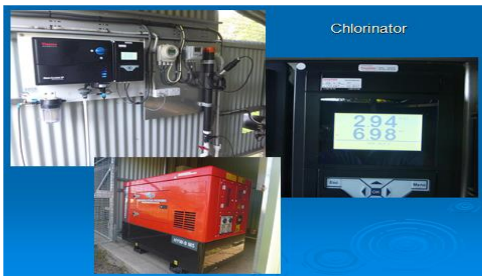
Figure 5.7: Facilities at the Bulgun Ck Chlorinator - Chlorine and Turbidity Analysers, Back Up Generator.
