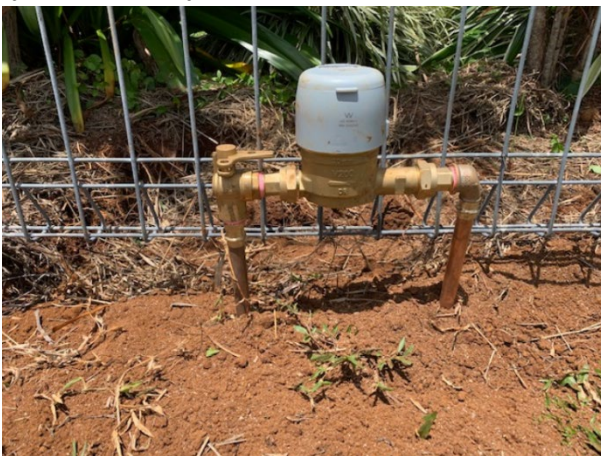
Photo above: A typical Honeywell V200 HT above ground water meter with in-built transmitter.
