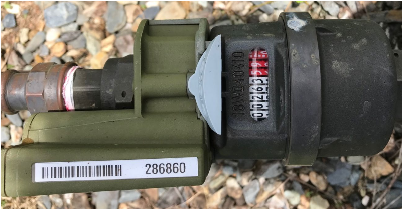
Photo Above: V100 meter with MRC transmitter showing 263.59KL.
