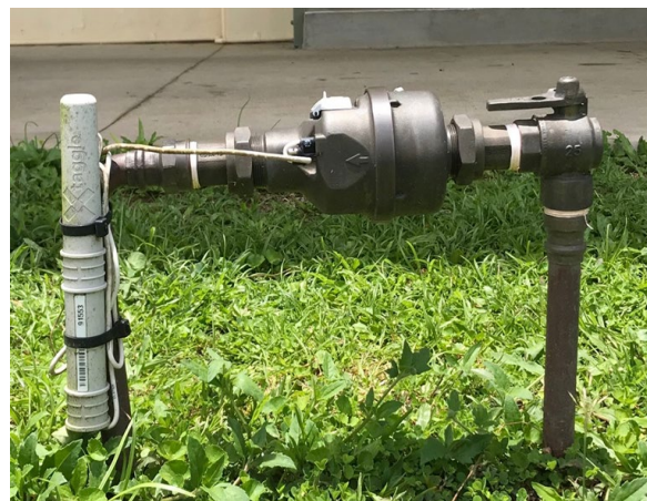
Photos above: (Left) Elster V100 meter with MRC transmitter. (Right) Elster V100 meter with HP transmitter
