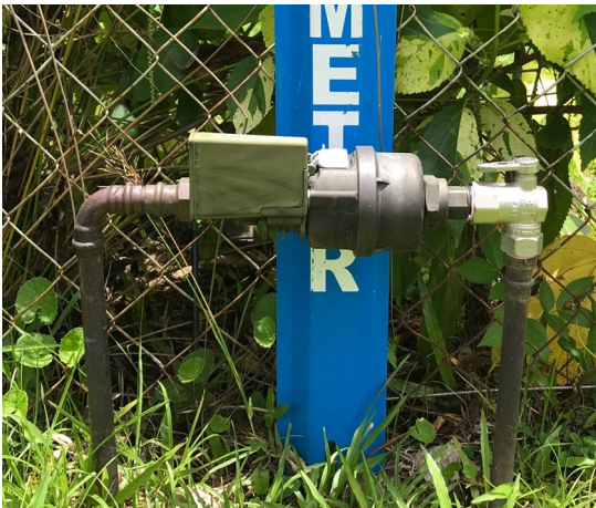
Photos above: (Left) Elster V100 meter with MRC transmitter. (Right) Elster V100 meter with HP transmitter
