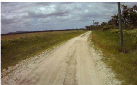
Thin gravel. Normal 10 to 30mm. Likely deterioration within 1 to 2 years.
