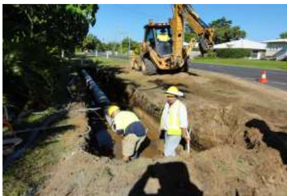
Replacing stormwater drains, Porters Promenade, Mission Beach.
